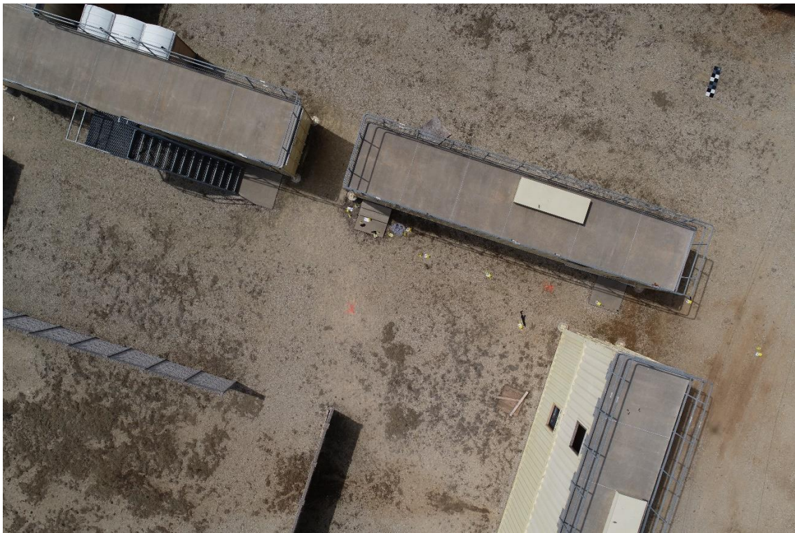
Figure 1. Vertical Aerial Photograph.
