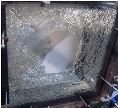
Figure 3: Broken Tempered Glass
